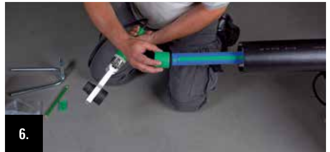
Directly after the removal of the welding device push the socket on the pipe end.
