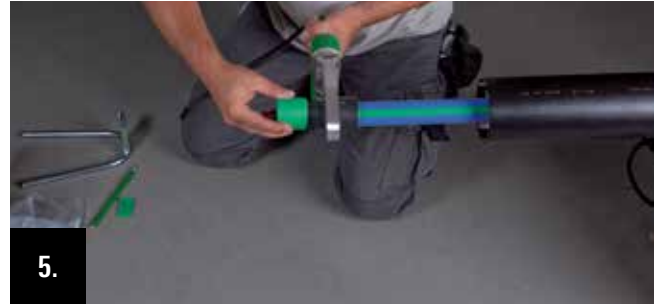
After the heating time pull off the welding socket and the pipe end from the welding tools.
