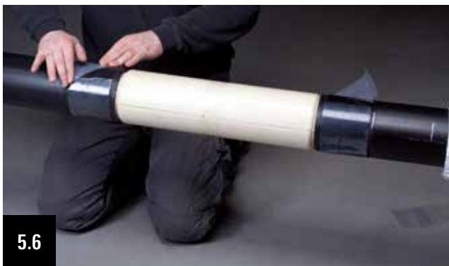
5.6 Wrap outwards the upper release liner on both sides in a 45° angle that the beginning of the film of both melting adhesive strips protrudes over the marking of the center distance.
