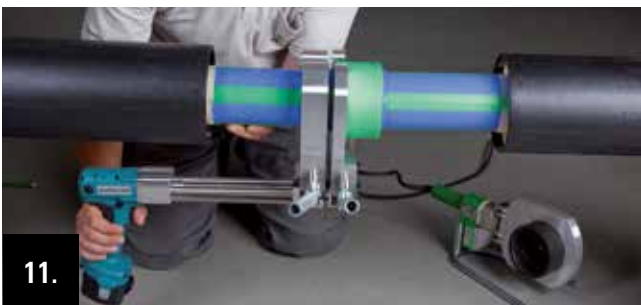
Press the pipe end, within the processing time, with the welding jig up to the end of the welding depth in the welding socket.
