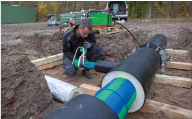
Timber must be removed after completion. Use rigid polyurethane foam boards or sandbags!
