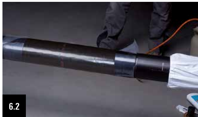
6.2 Gently heat the end of the shrink film at the bottom side – like the melting adhesive strips. Then wrap the heated part around the pipe and press it tight in the overlap area.
