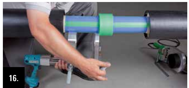
Open the clamping jaws of the welding jig as far that the welding jig can be removed sidewise or downward from the connection.
