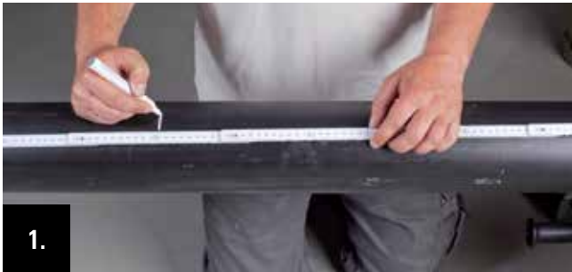
1. Measure the pipe length and mark on the casing pipe.
