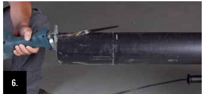
6. Slit the casing up to the PUR-insulation layer with a customary handsaw for plastic.
