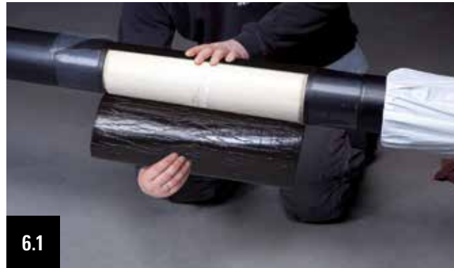
6.1 Remove the release liner at the bottom of the casing shrink film. Center the film over the PUR-insulation sleeve in a 90° angle to the pipe axis and wrap closely around the PUR-insulation sleeves. A sufficient overlap of the shrink film of at least 10 cm is important. On both ends the shrink film must overlap the casing pipes with at least 2.5 cm.
